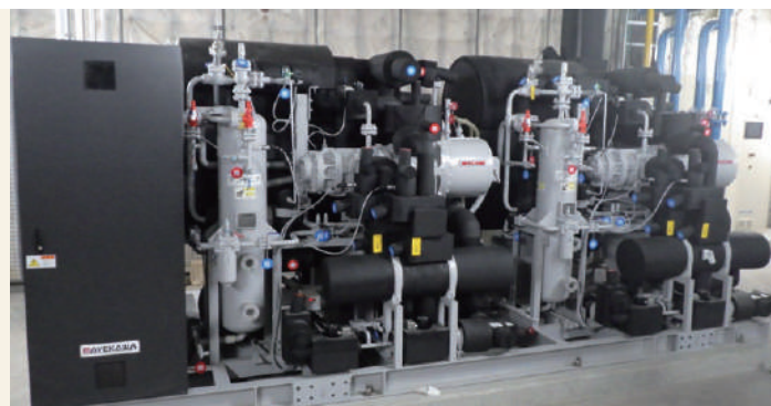
CFC-free refrigeration equipment used by Kyokuyo Akitsu Reizo Co., Ltd.
